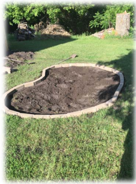
ADDING PAVERS AND MULCH, SHAPING DEPRESSION.
