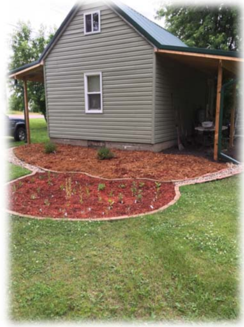
INSTALLING RAIN GUTTERS AND DOWNSPOUTS, CREATING FLOW PATH TO RAINGARDEN.
