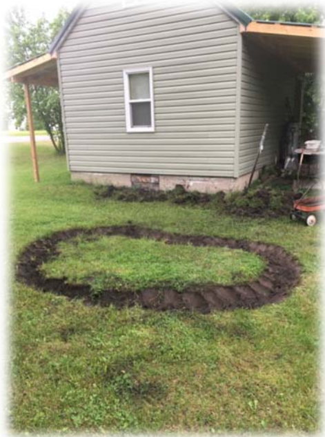
EXCAVATING ROUGH SHAPE OF THE RAINGARDEN.
