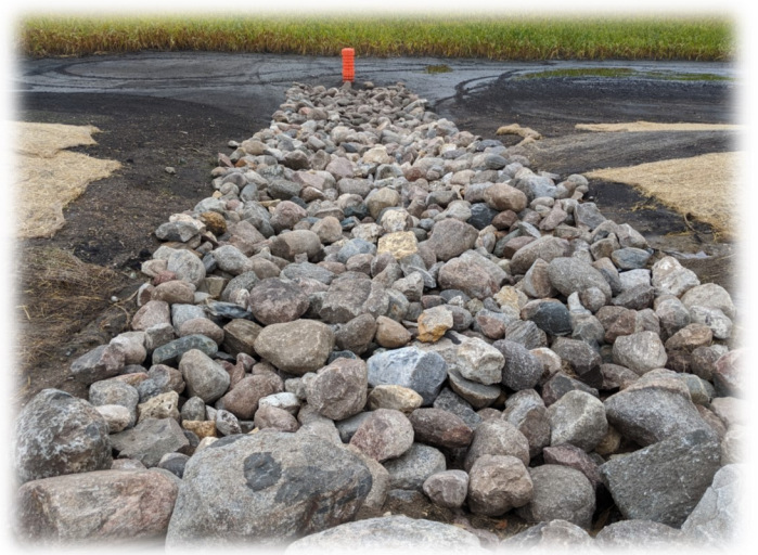
COMPLETED ROCK LINED CHANNEL.
