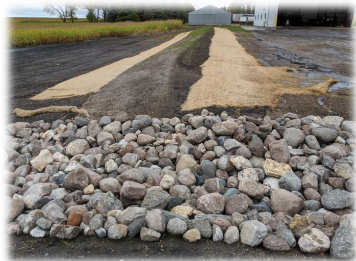
EMBANKMENT NORTH OF CHANNEL, WITH VEGETATION BEGINNING TO GROW.
